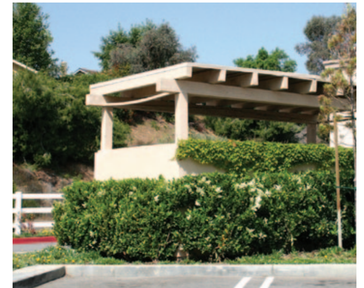
SCREENED TRASH ENCLOSURE
