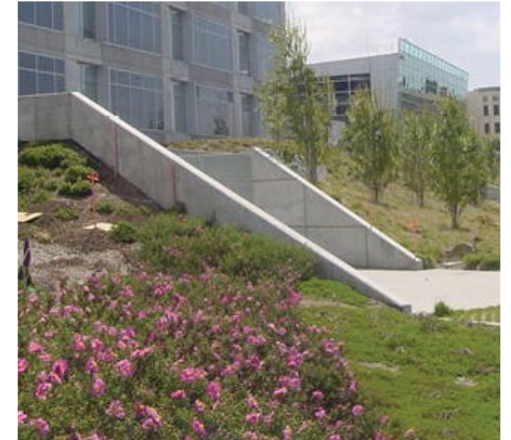
SCREENED LOADING AND DELIVERY AREA
