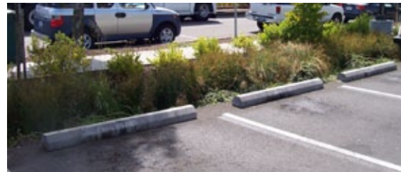
BIOSWALE AT PARKING LOT
