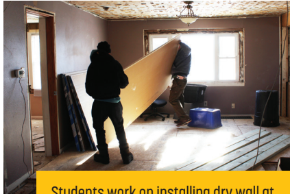
Students work on installing dry wall at the Community Build home. Learn more at www.medcoiowa.org/marioncommunitybuild
